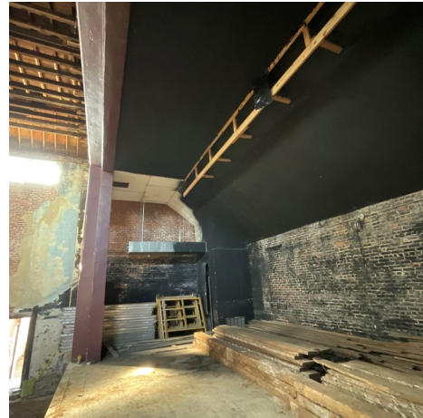
Figure 6 – Ceiling at Stage
