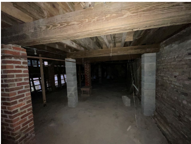
Figure 9 – Basement (Looking North)
