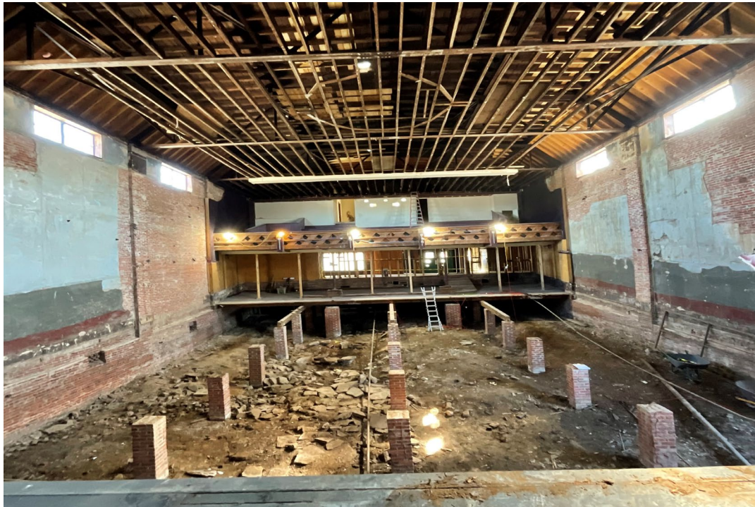
Figure 1 – Theater Space (Looking East Towards Balcony and Lobby)
