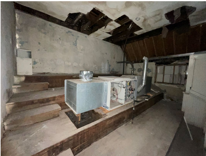
Figure 7 – Mechanical Unit at Balcony and Clerestory Window
