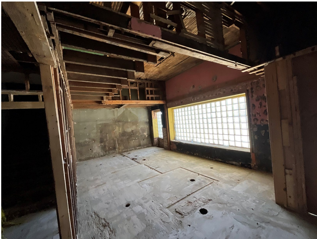
Figure 4 – Lobby (Looking North)
