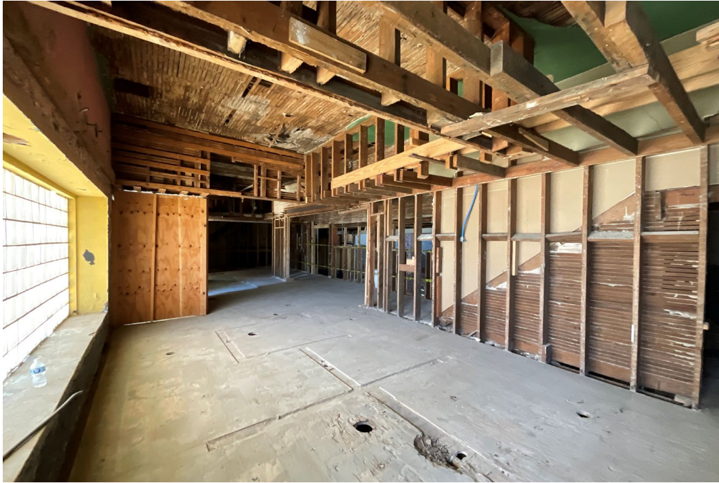
Figure 3 – Lobby (Looking South)
